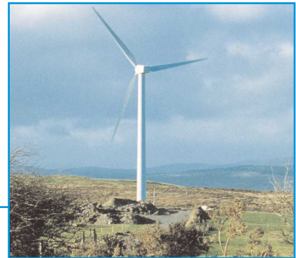
...and new wind turbine in Cork
